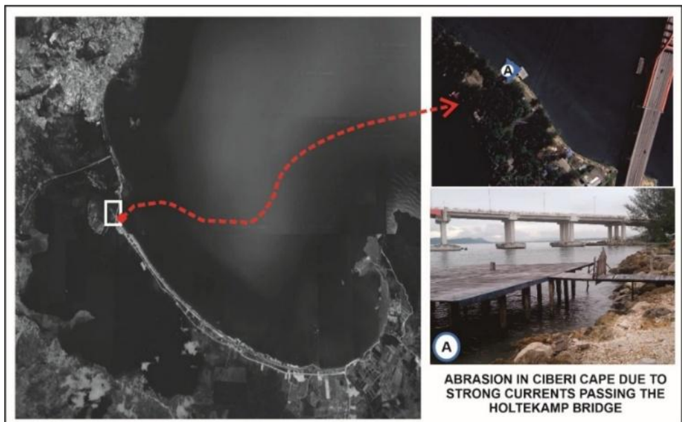
Figure 10. Abrasion location in Ciberi Cape due to Strong Currents Passing the Holtekamp Bridge
