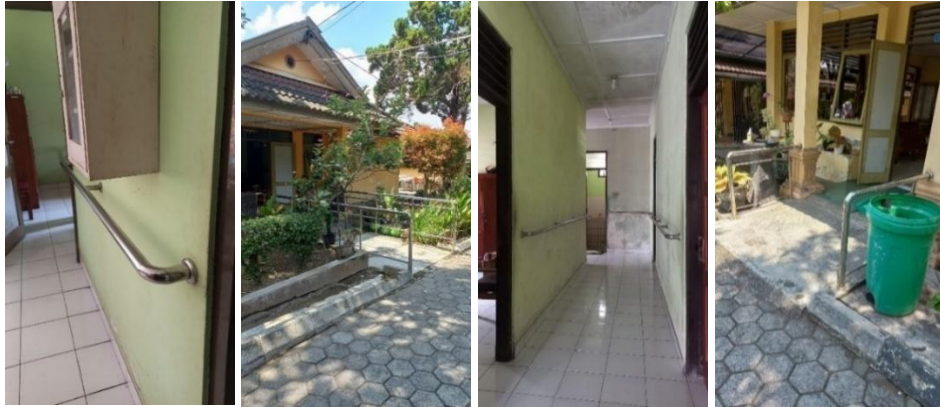
Figure 5. Hand railing and ramp in the BPSTW
