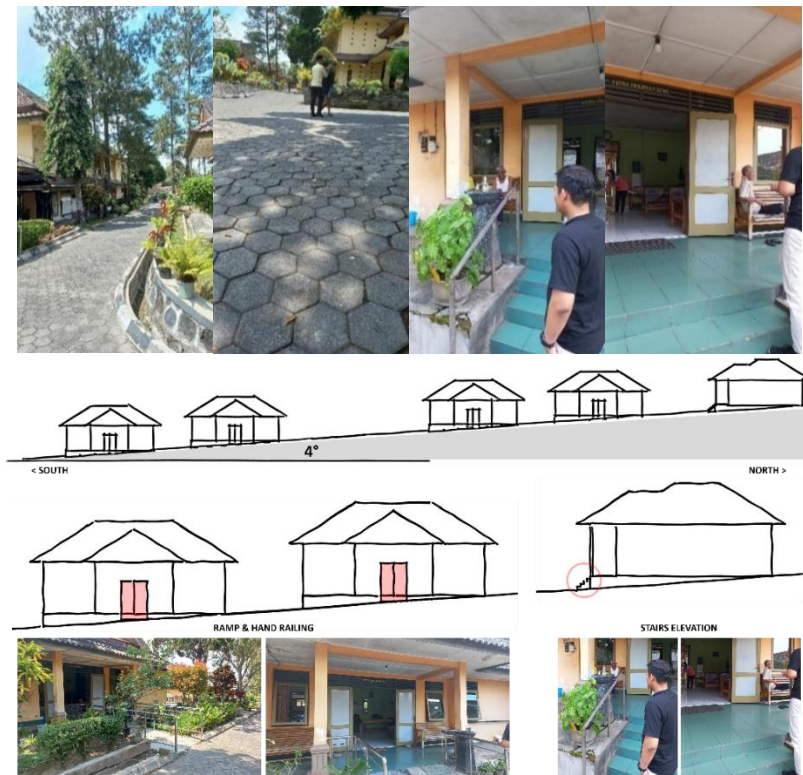
Figure 8. The ground level is getting higher to the rear and access stairs at guest houses
