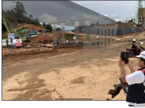
Fig. 1. Augmented Reality on road and bridge infrastructure in Indonesia's New Capital City Construction
