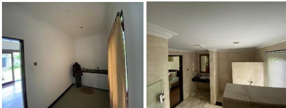
Gambar 2. Eksisting Fasilitas Interior Suite Room
