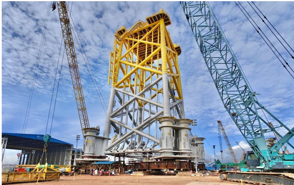
Figure 1. Construction of Offshore Wind Farm Jacket (Source: Changhua Project in Batam)
