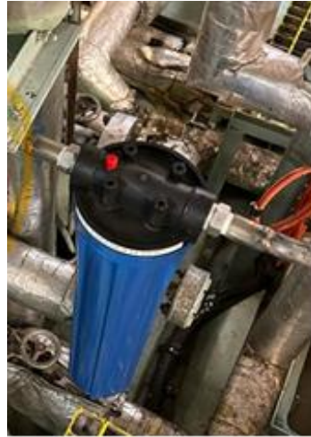
Figure. 6. Installation of a New Water Filter
