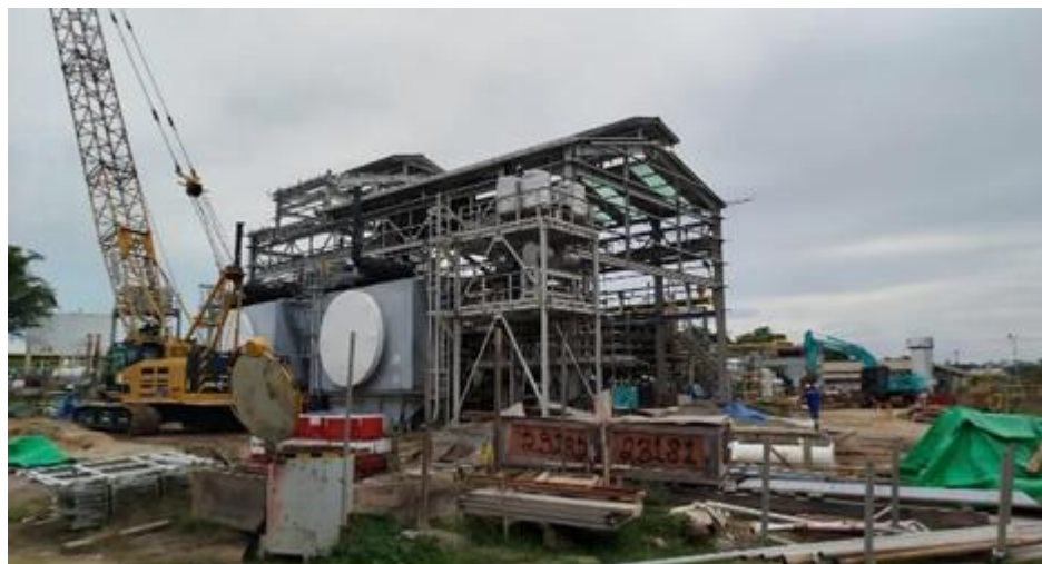
Figure 1. Installation Progress of the ULP Compressor
