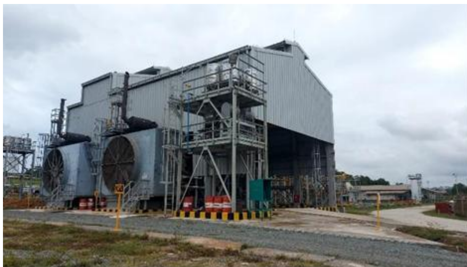
Figure 2. Completed Installation of the ULP Compressor
