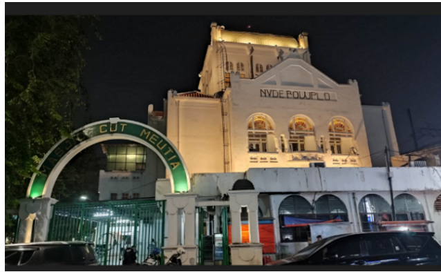
Fig. 4. Cut Meutia Mosque is visible from Jl. Taman Cut Meutia. Source: Author, 2024
