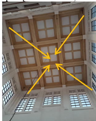
Fig. 15. The interior of the roof is covered with a ceiling with a square pattern. Source: Author, 2024
