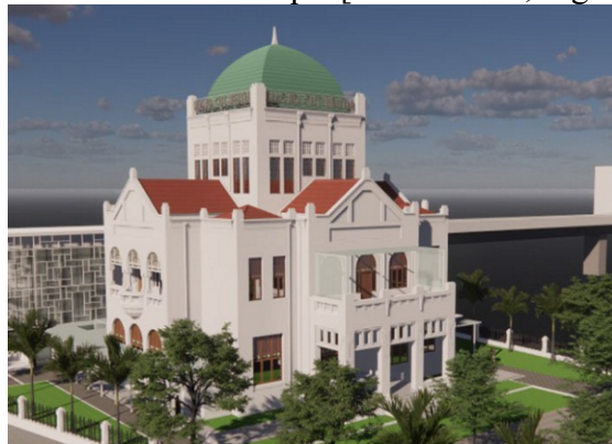
Fig. 5. The shape of the roof of the Cut Meutia Mosque.
