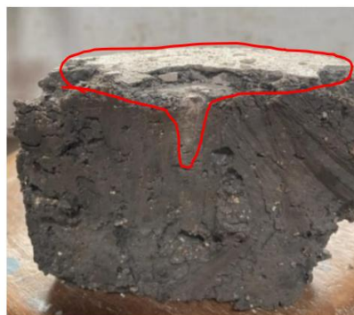
Figure 5. A layer of cement paste on the surface of the soil sample at Sta.37+850 source: Author's Data, 2022
