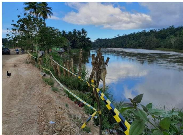
Figure 2. Temporary repairs of the landslides by placing a recess made of wooden stakes This section is a vital segment because there are mining and processing of nickel ore.
