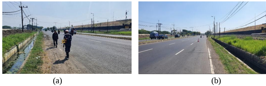
Figure 2. (a) Existing Condition on West Side KM 31+450 (b) Existing Condition on East Side KM 31+450
