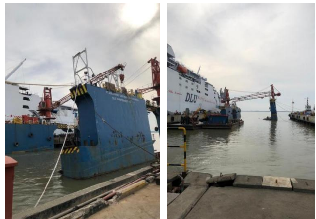
Figure. 1 The Damaged of Floating Dock
