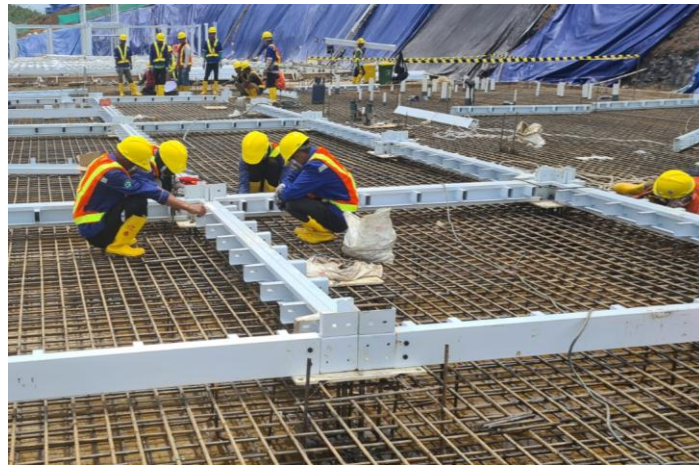
Figure 2. The process of installing the foundation
