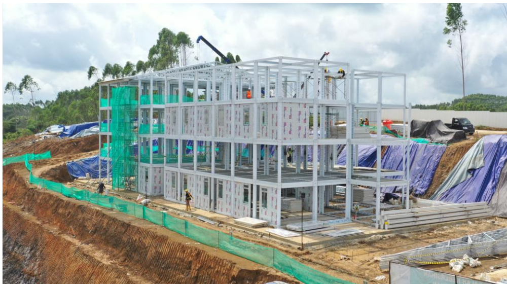
Figure 1. The process of installing the Modular Box
