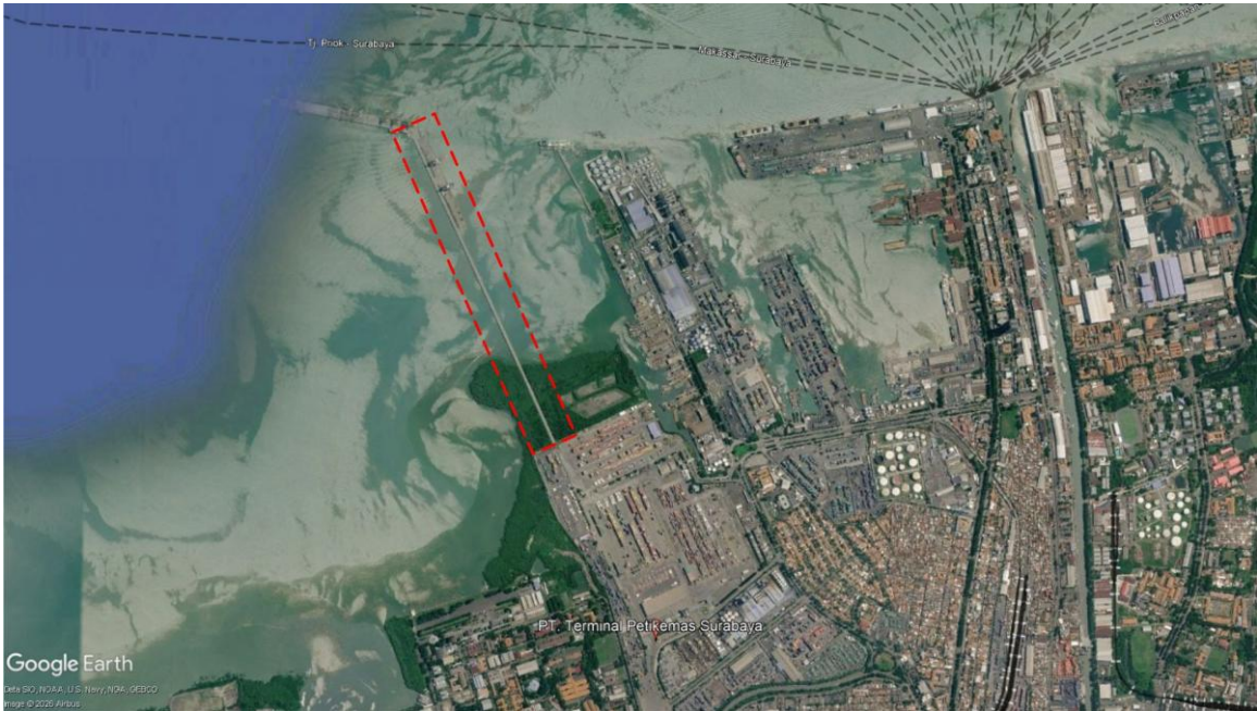
Figure 2. Location of Access bridge at PT Terminal Petikemas Surabaya.
