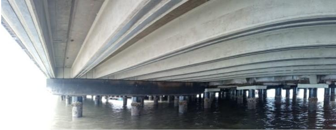
Figure 1. Access bridge at PT Terminal Petikemas Surabaya.
