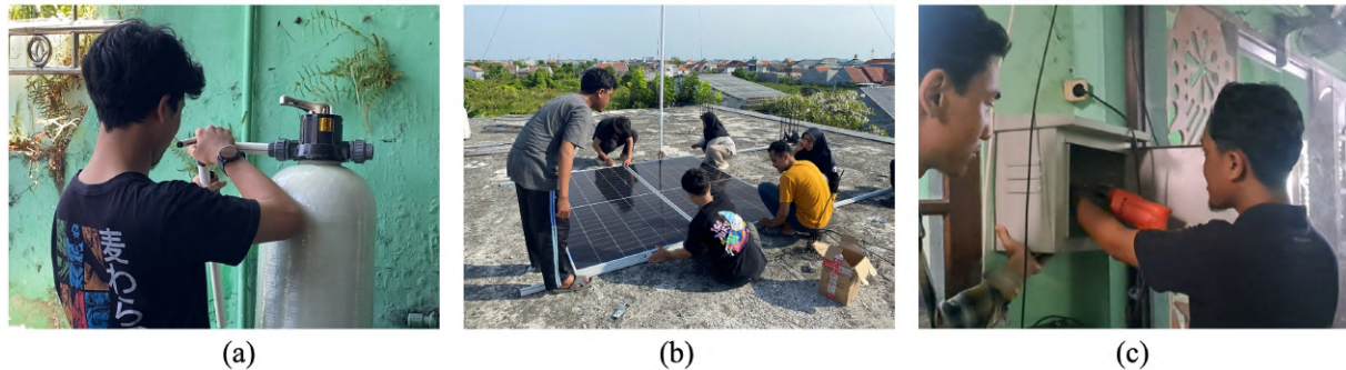
Gambar 8 Pemasangan (a) Water Filter (b) Panel Surya (c) Panel Box .
