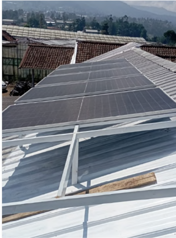
Gambar 10 Instalasi Panel PV Bifacial di Atap Gudang Cold Storage .
