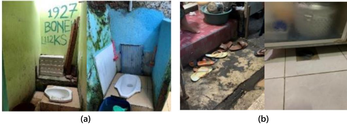
FIGURE 1. Existing Healthy Latrines; (a) Toilets, (b) Septic Tank Location)
