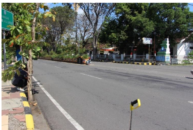
Figure 6 The type of road pavement on Yos Sudarso Road
