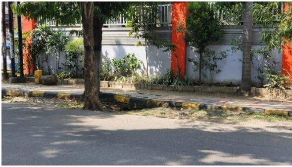
Figure 3 Cleaning up the trash is necessary to optimize the water flow into the side channels.
